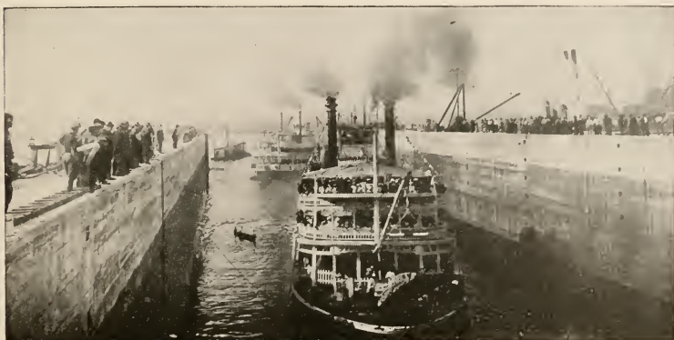
The colossal Keokuk lock in the Mississippi as wide as those at Panama and with a higher lift than any one lock on the Isthmus.
