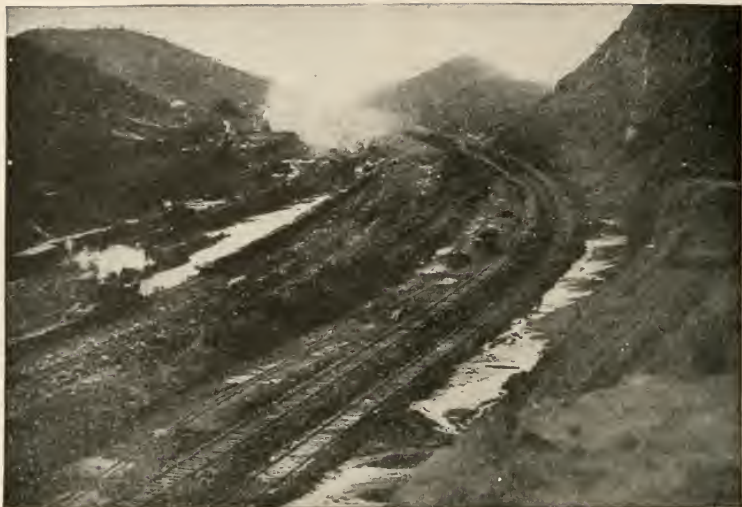
The mighty cutting through the Culebra mountain shown here is one of the wonders of the world. The engineers literally moved mountains. Altogether 300,000,000 tons of earth were removed for the canal.
