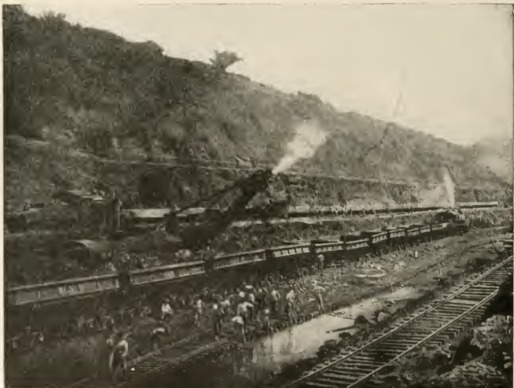
This is another part of the cut through the Culebra mountain. To blast away the rock more than a million cartridges were exploded in a year, and the removal of the material excavated is no less wonderful than the excavation.
