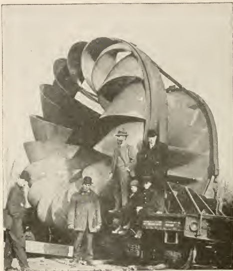
One of the thirty titanic turbines of the Keokuk water-power plant, several times as large as any ever built before. It weighs several hundred thousand pounds and revolves with the power of ten thousand horses.
